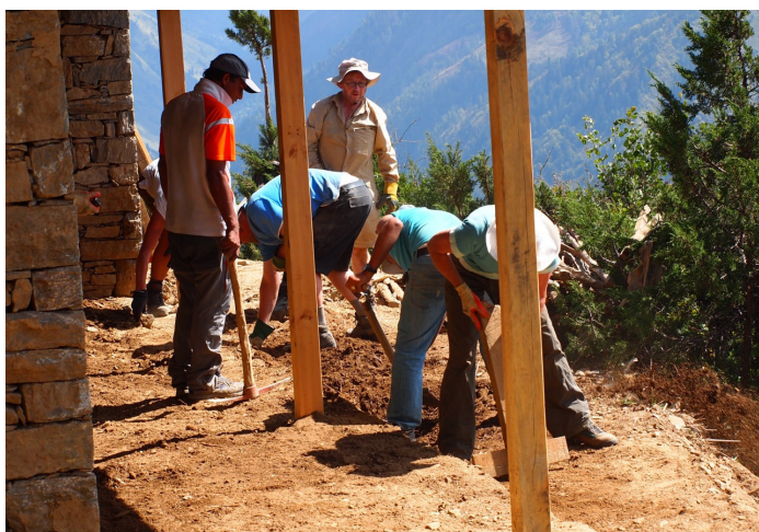
Helping construct the clinic in October 2010
